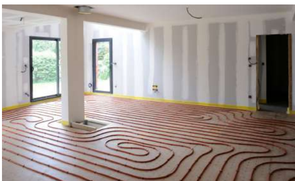
Plancher chauffant
